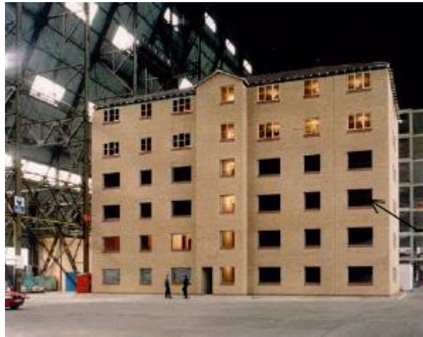
Figure 12. 6 storey TF2000 timber frame test building in BRE hangar at Cardington [45]
